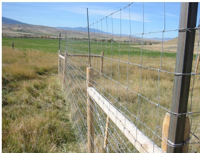
FIGURE 1. Mesh fence extension on top of existing livestock containment fence
